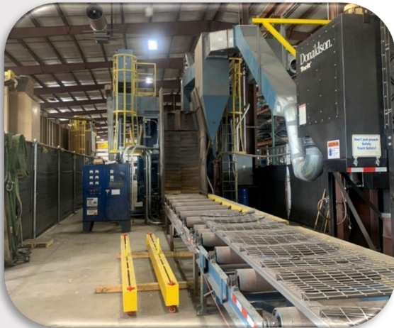
6-Wheel Blastec Shot Blast Machine – Conveyer/Crane Fed
