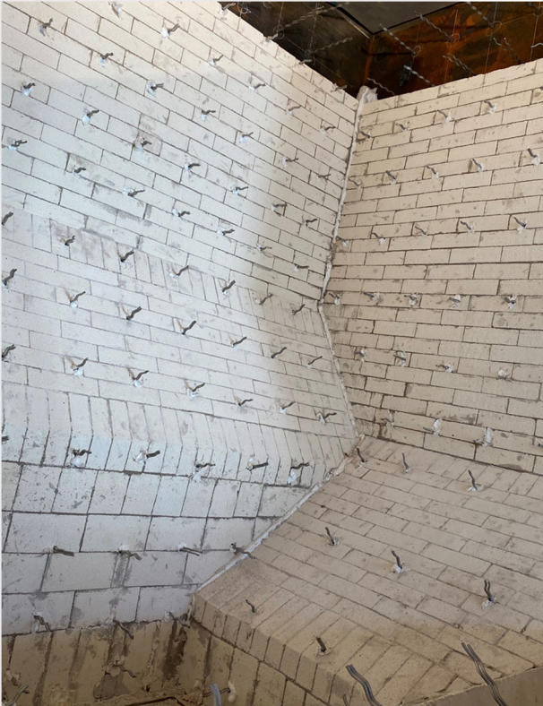
2 nd Layer of insulation brick in downcomer.
