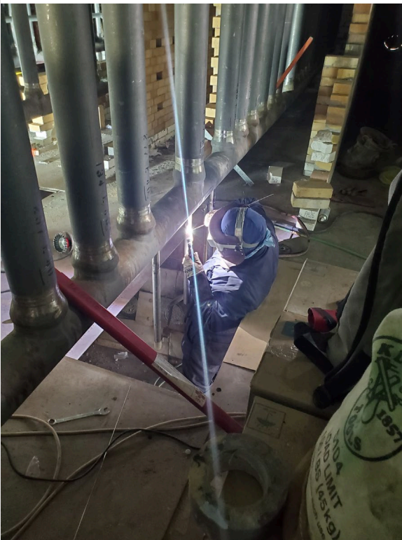
AWVI TIG welding on Harps – drain nozzles and TI sleeves.
