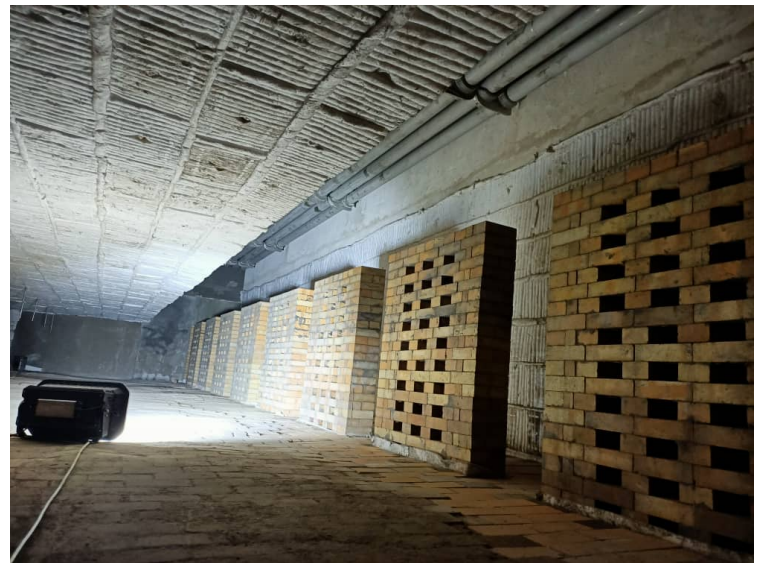
Completed Transition Roof using Z-Blok modules with brick Baffle Walls completed
